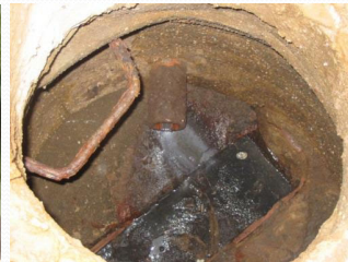
Gray/black staining in a storm sewer
