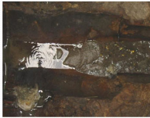
Sanitary debris in a storm sewer
