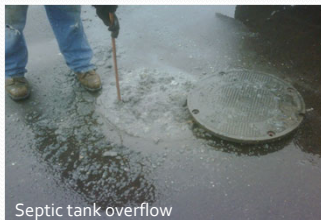
Septic tank overflow
